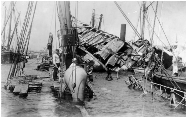
View of Wreck of "Maine" from aft. 19 - 9 - 21.
